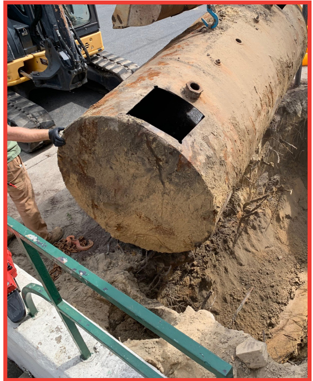
Underground Tank Removal
