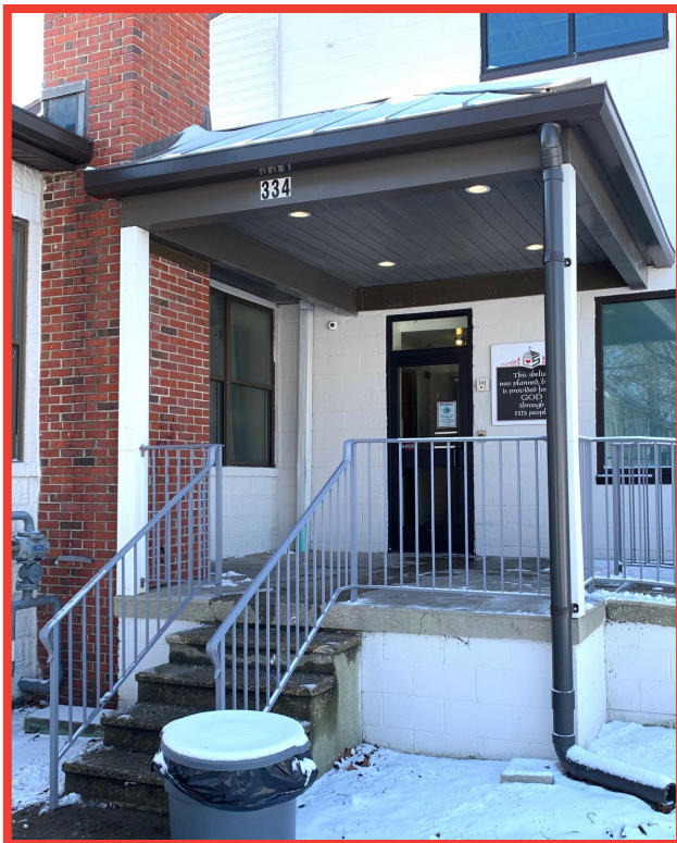
Front Porch - New Gutters/Downspouts
