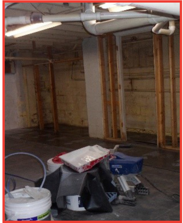
Mold Remediation in the Basement
